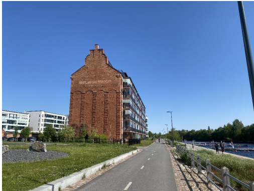
Vaasa mill. The first part of the mill was completed in 1924. In later years, the mill has been expanded four times. The building was converted into a modern residential building in 2018 preserving one end of the old mill and rebuilding the rest.
